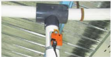
125 mm Drop Point With Motor Valve
